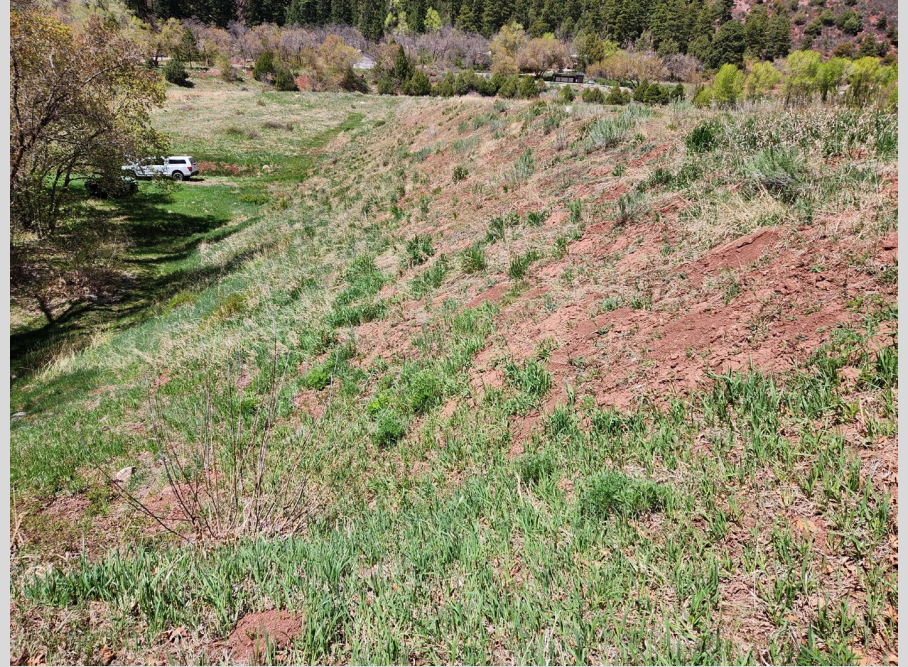
Downstream Slope from Left End
