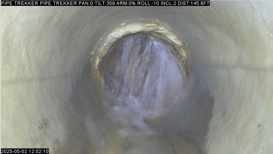
Elbow – Note Leakage
