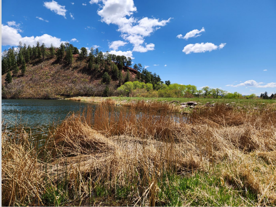
Spillway Approach Area
