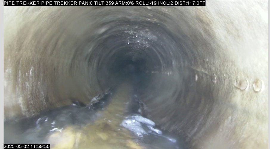
117.0 Ft. – Hydraulic at Grade Change
