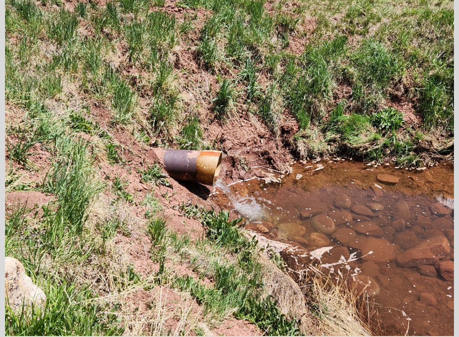
Outlet Following Inspection
