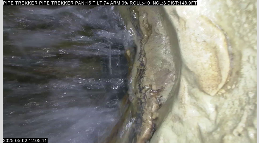
Leakage at Elbow – Epoxy Repairs to Liner During 2013 Install
