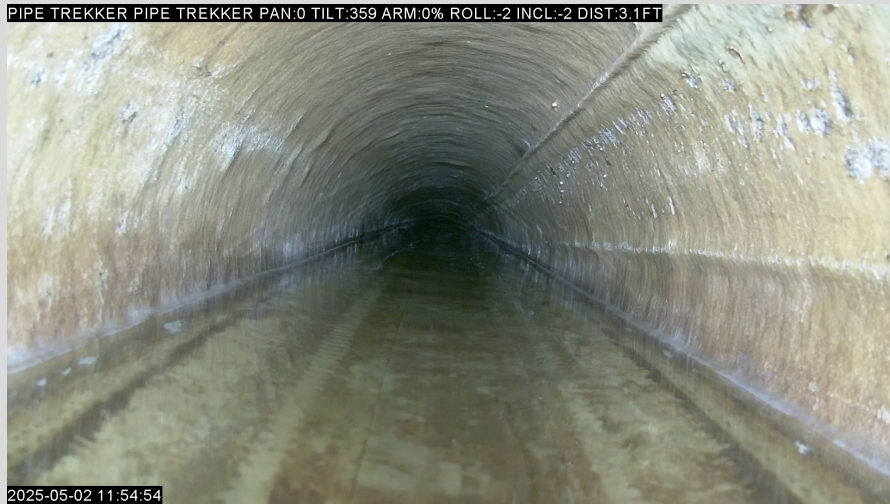
CIPP Line WSP from Near Outfall
