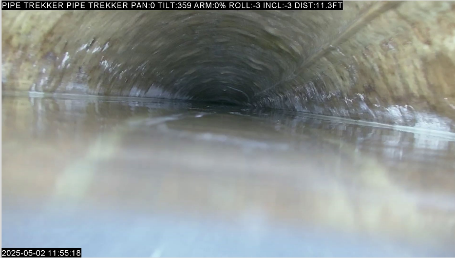
11.3 Ft. – Incline -3 deg., Poned Water to Spring Line
