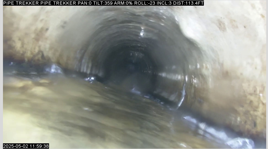
113.4 Ft. – Protrusion in Liner at 1 o'clock
