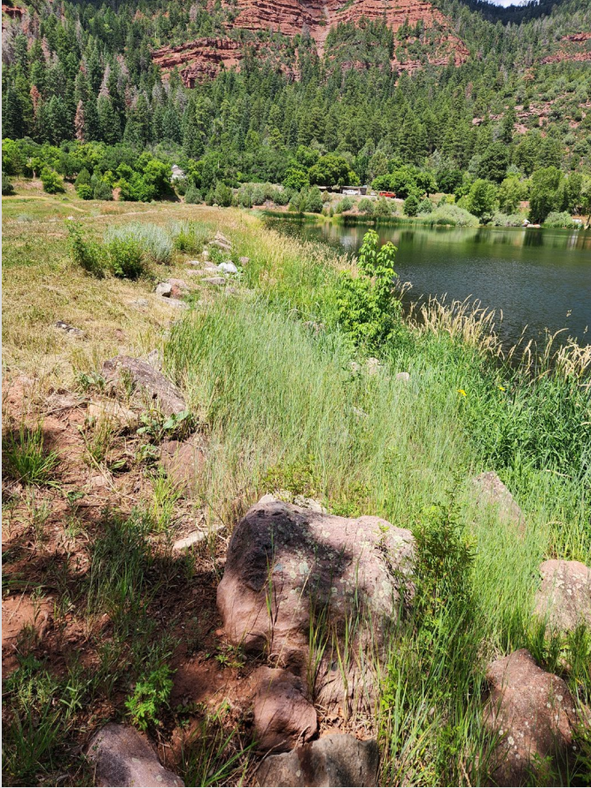
Upstream Slope from Left End
