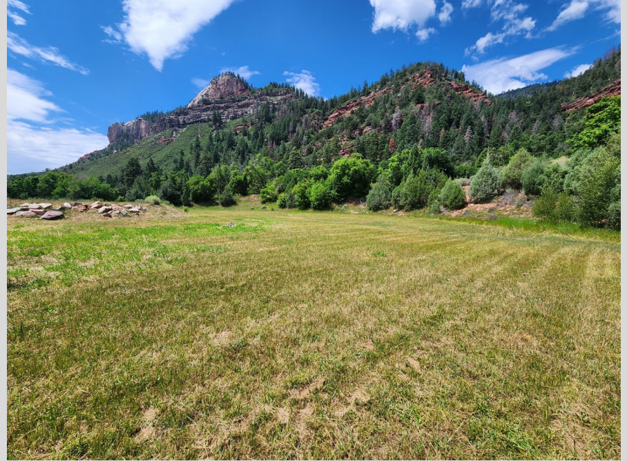
Spillway Channel – Looking Downstream
