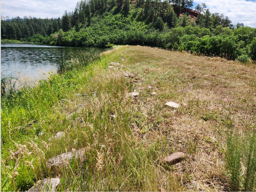
Upstream Slope and Crest
