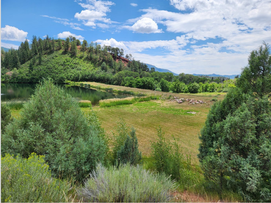
Spillway Channel – Upstream End
