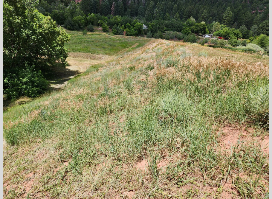
Left Groin and Downstream Slope
