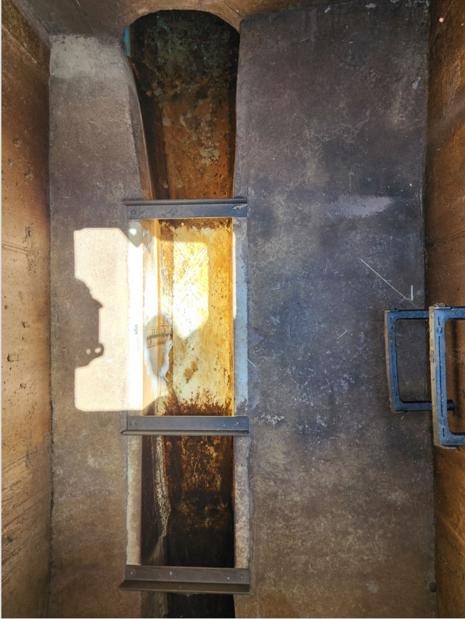
Flume Inside Vault
