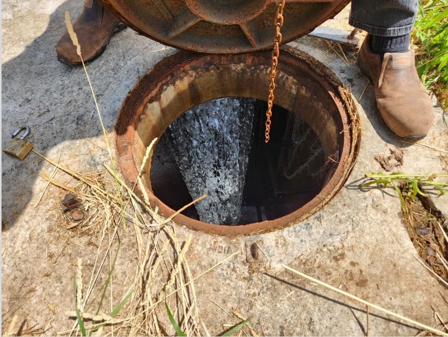
Flow Over Gate Inside Vault
