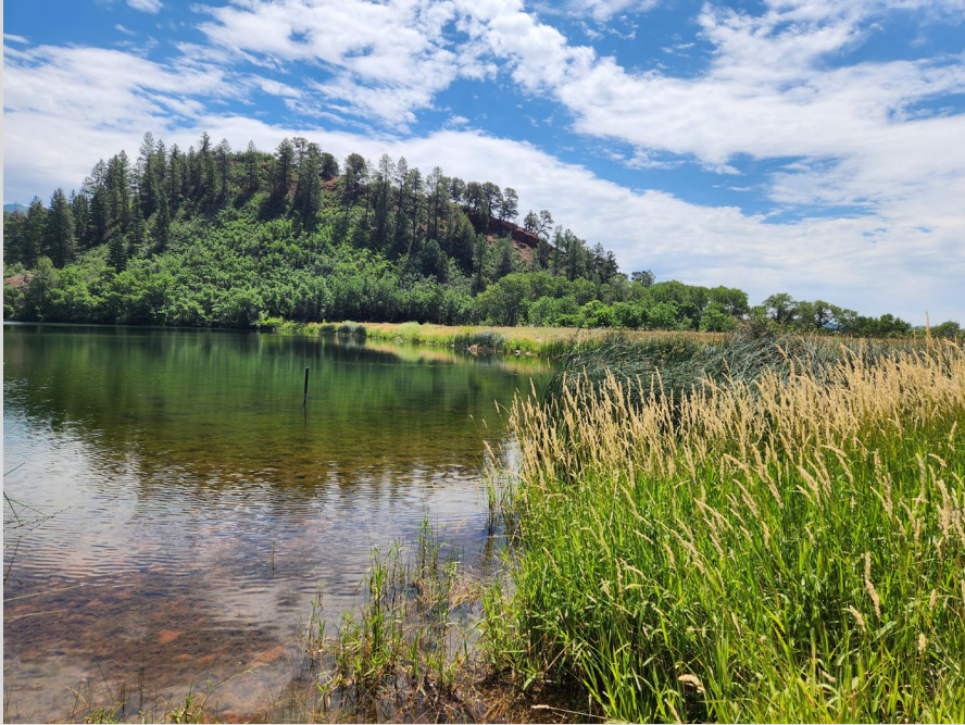
Looking at Upstream Slope from Spillway
