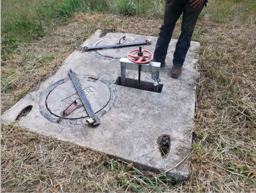
Flume Vault in Spillway Channel
