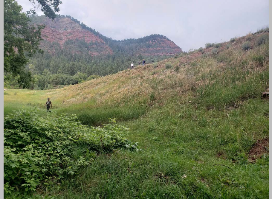
Toe Area from Near Left End of Embankment
