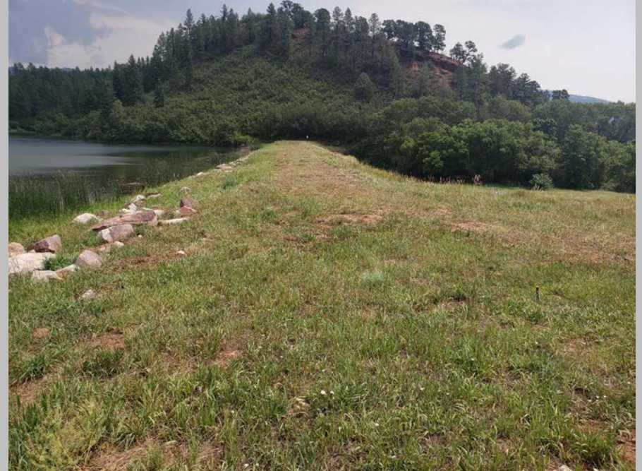
Crest from Right End of Dam
